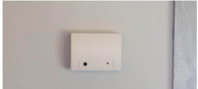
**Step 5:** Due to the advanced false alarm detection on the glass break sensor it may be unlikely to trip using substitutes such as keychain noises or glass break noises on a phone or speaker. You can test to make sure the glass break is detecting audio by making a high pitched noise next to it - such as clapping. The red LED should flash indicating audio being detected.
